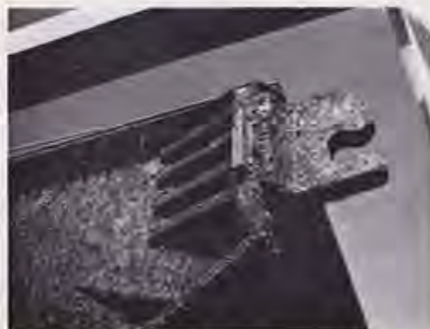
Fig. 32 Shellfishes attached near hinge bracket (Koyagi)
