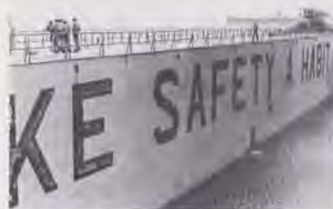
Fig. 12 MSHI repair dock gate
