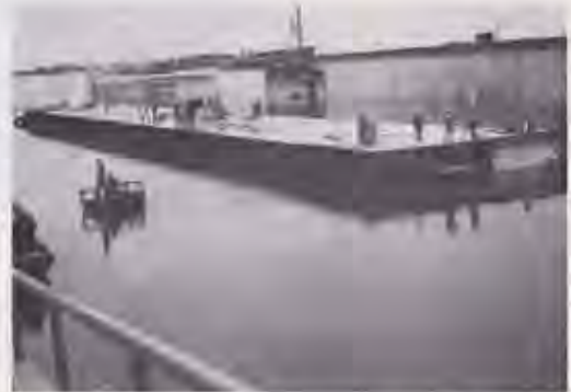
Fig. 18 Gate afloat on water surface for installation (MSHI)
