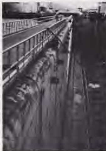
Fig. 10 Koyagi repair dock gate
