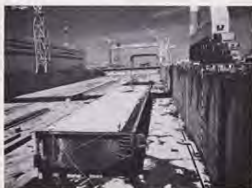
Fig. 31 Gate dry-docked for maintenance (Koyagi)
