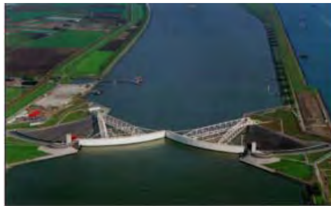
Fig.-1 Image of Horizontal Sector Gate
